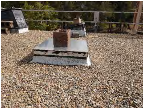
RF01- Roof Flashing
