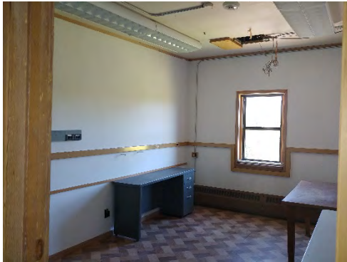
Composite drywall w/joint compound walls, ceilings throughout all 3 floors (CDW01, 02, 03, 04) and MA02 - walls w/wallpaper
