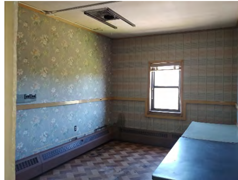
Composite drywall w/joint compound walls, ceilings throughout all 3 floors (CDW01, 02, 03, 04) and MA02 - walls w/wallpaper
