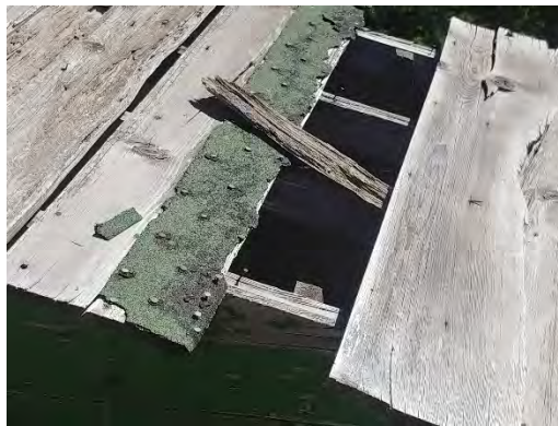
RSG02-asphalt roofing shingles on wood storage shed
