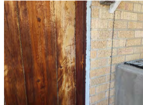
CK03- exterior Storage Rm, door frame
