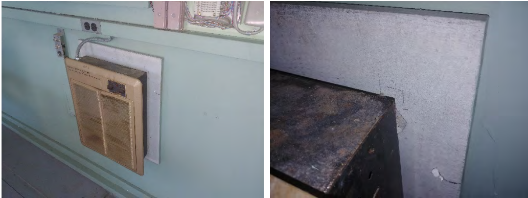
CB01- cement board behind wall mounted heaters
