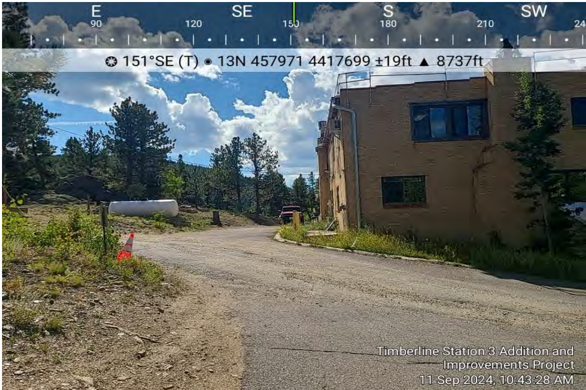
Photo 5. North end of the Fire Station and circular driveway that would provide construction access.
