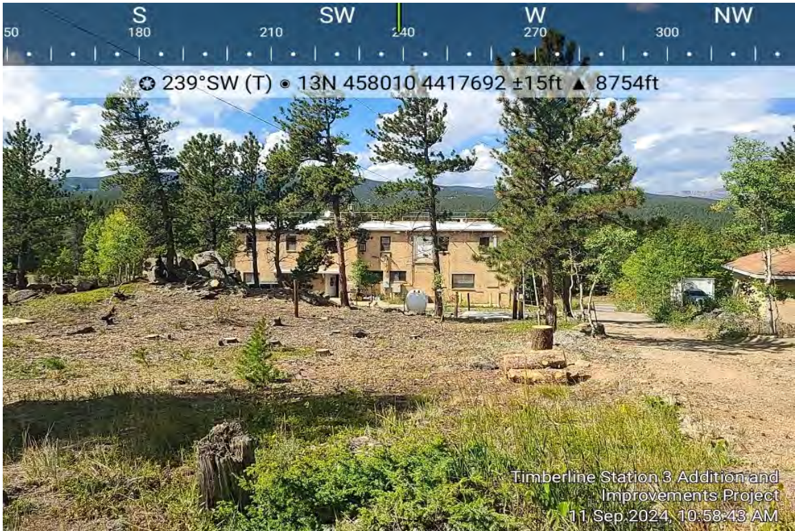
Photo 7. Rear of the Fire Station and disturbed area where additional staging would be, if needed.
