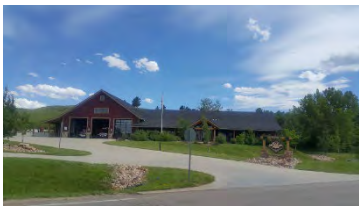
Rocky Mountain Fire Station No. 6, Eldorado Springs
